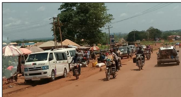
Figure 7: Poorly maintained Road in Otukpo Town
